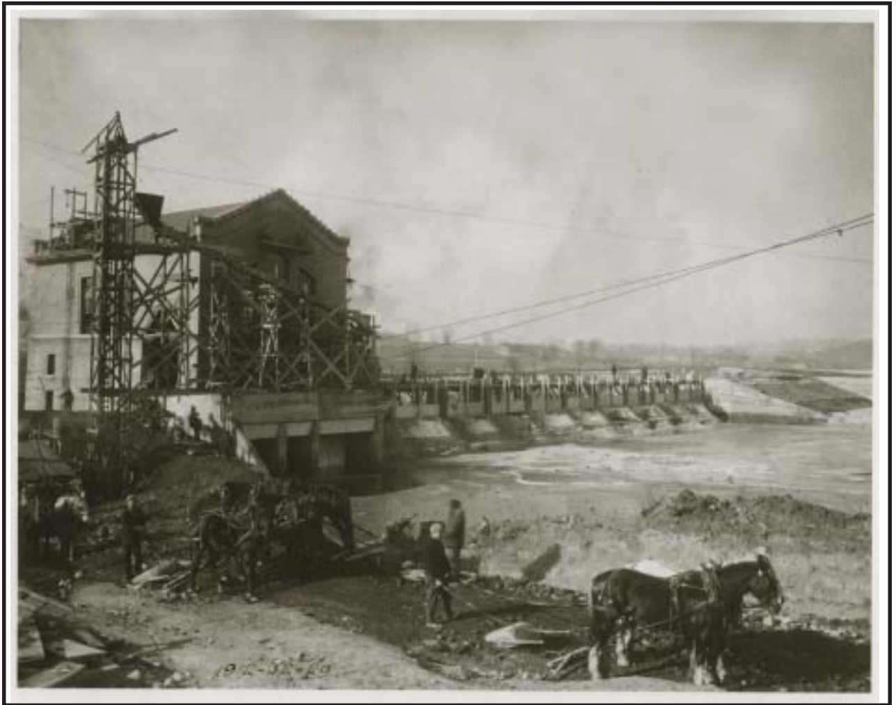
Construction of Barton Dam - 1927
