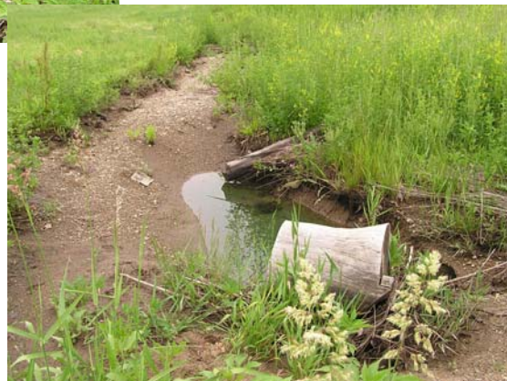
Photos 4 and 5. Drainage ditch on south end of project where it emerges from culvert. 6-10-09.
